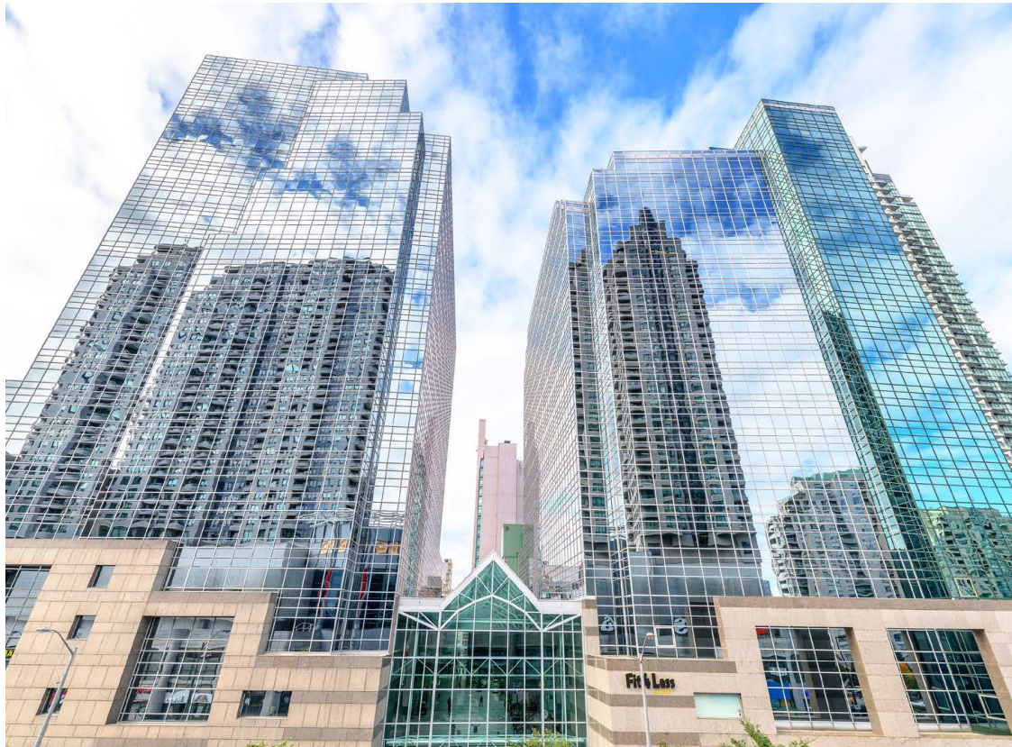
North York Centre 5140 and 5160 Yonge Street, Toronto, ON
